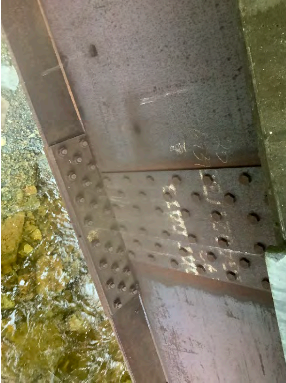
Left Bank Abutment when facing downstream
